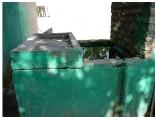
A pila (concrete structure at most homes to store water while not running the tap, common in most Central American countries)
