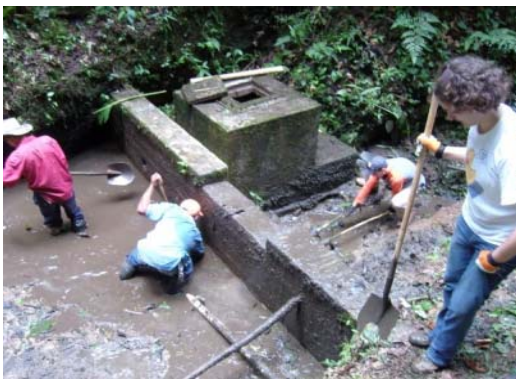
Dam where spring collects – source (beginning of system)
